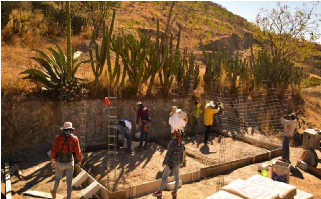
Photo: rebuilding the community
