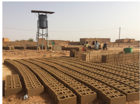
Photo: Water tower and bricks for construction.
